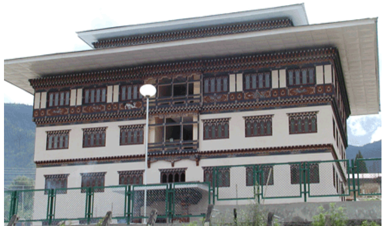
The Bhutan Integrity House, Kawangjangsa, Thimphu
